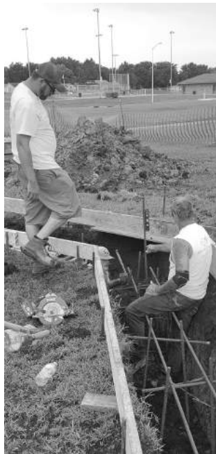
Loren Shriver and crew from A-1 Concrete Grinding were setting forms last week, preparing to pour concrete footings for the Martin County Veterans Memorial wall in Fairmont. (Submitted photo)
