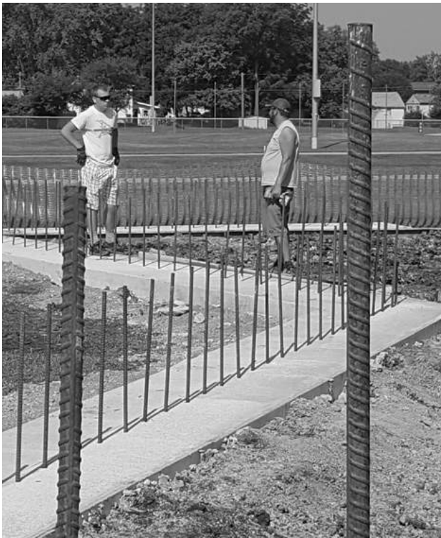
A-1 Concrete Grinding employees strip forms from concrete footings that were poured and re-rod prepared for the concrete wall in preparation for granite memorial wall at the Martin County Veterans Memorial in Fairmont last week. (Submitted photo)
