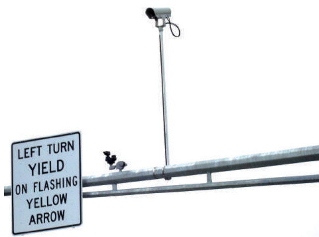
VEHICLE DETECTION CAMERAS are now installed at the traffic signals on the newly reconstructed Highway 15/State Street highway.
